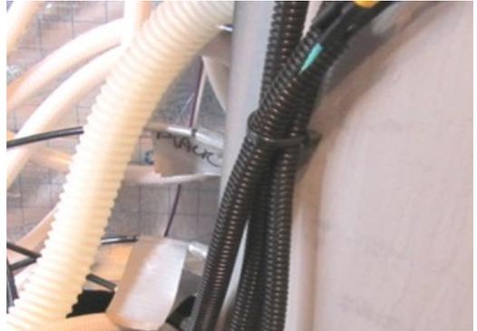
**Fig. 18 A** IP 66 wire pairs and 12V supply wires sheathed over and tie wrapped
